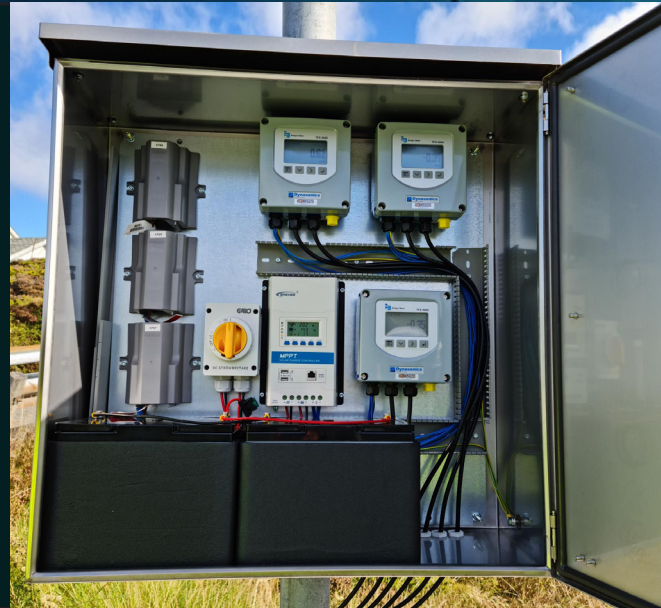
LEAKCELL® model LC322 with three ultrasonic flow meters, battery bank, charging regulator and web portal mobile transmitters
